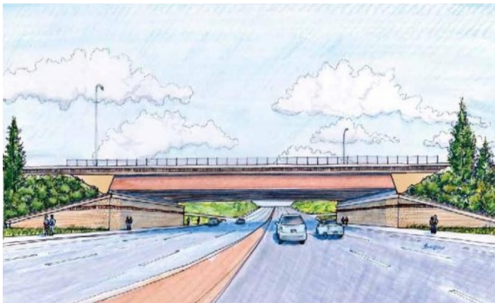
Hampden Avenue bridge over Wadsworth Boulevard, looking south, with wider medians and no center pier.
