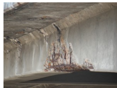
Current bridge condition over Wadsworth Boulevard.
